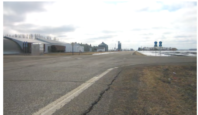
Looking South on County Road 2 at the Intersection with County Road 1
