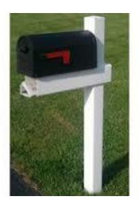
**Prohibited:** Mailboxes supported by structures such as non-breakaway masonry columns, railroad ties, tractor wheels, plow blades, concrete barrels, and any other non-breakaway style support systems are not acceptable.
