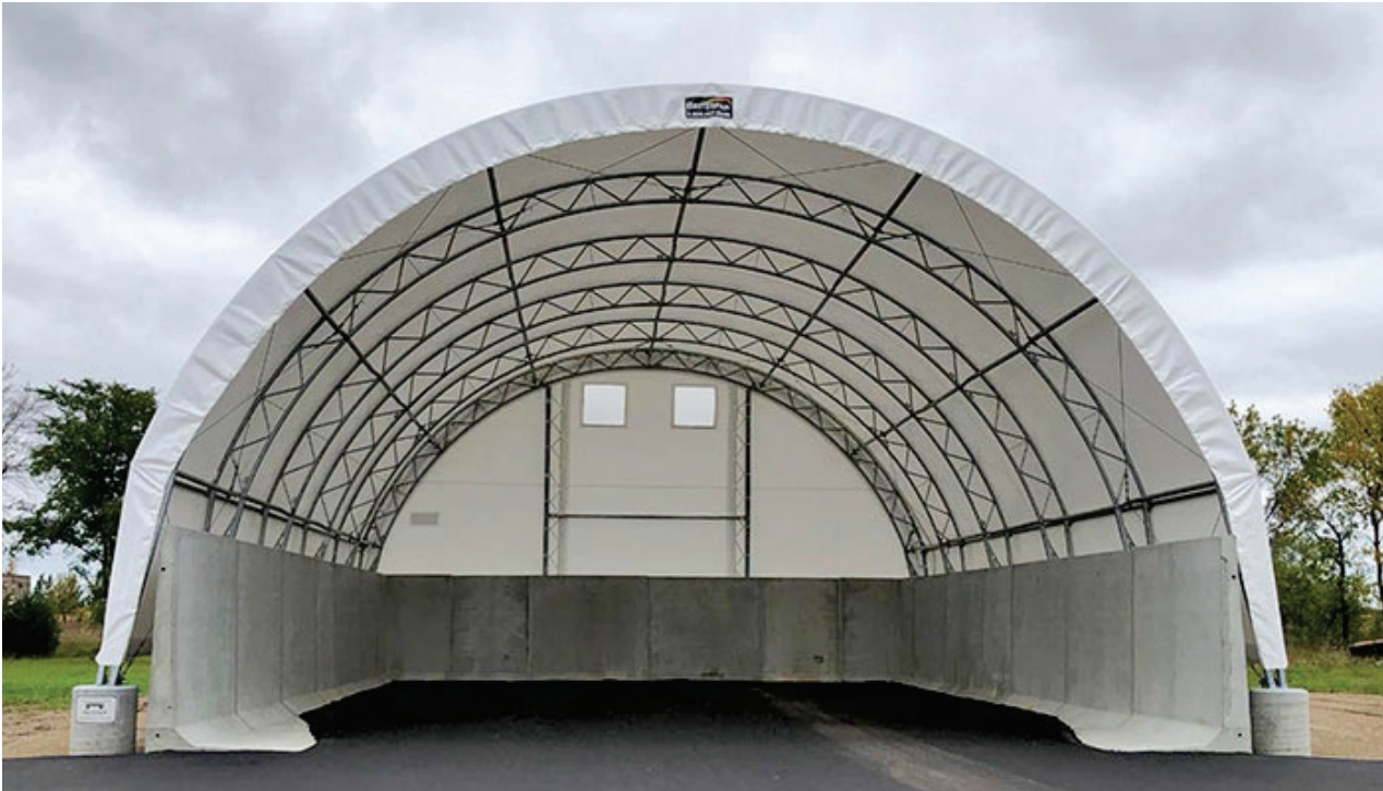
Example of Similar Salt Storage Building
